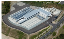
71 12GB10872 Data Center [Matsue Data Center Park:Outside-air-cooled Container Data Center] Matsue Data Center Park is Japan's first container data center offering the low-cost, high density, and scalability for the demands of the cloud computing era.
