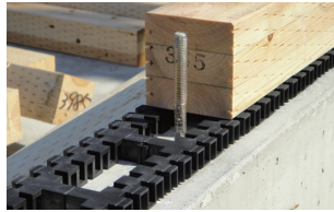
Underfloor ventilation system [Joto Kiso Packing Method] JOTO TECHNO CO.,LTD. (Award number:26L221506)
