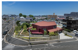
Office architecture [YUKI office] UENOAarchitects / YUKI / Hakko Construction Co., Ltd. (Award number:26G141005)
