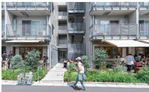
apartment complex [KOENJI APARTMENT] JR East Urban Development Corporation / Open A Co., Ltd. / DAIICHI KENSETSU Co., Ltd. / Mamekurashi (Award number:26G130918)
